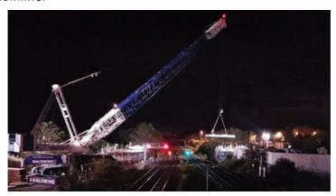
The £2.5m project will involve reinstating some 500m of missing embankment, track and bridge. The first phase of the work on 3rd September saw two steel beams being put in place for the new bridge, with the decking being added later.
